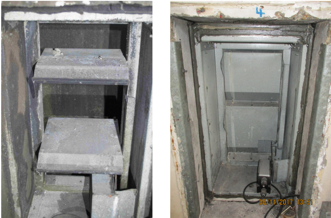
Figure 60.3 – Examples of dampers in an open and closed position
